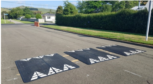
Figure 16 Example of Speed Humps/Cushions
